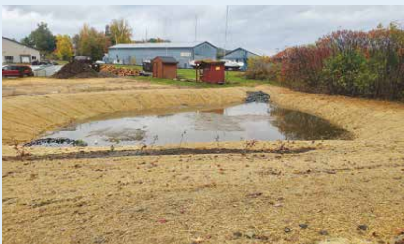
New gravel wetland swelling with stormwater immediately after construction.
