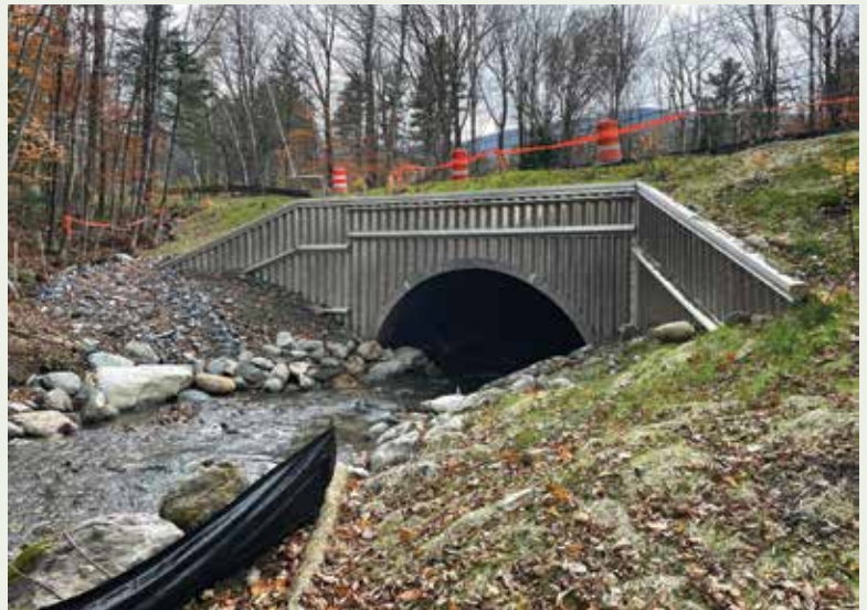
Before (top) and after the Lockwood Brook Culvert project
