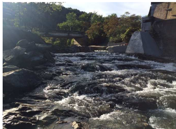
Hyde Dam site after removal (WRP)
