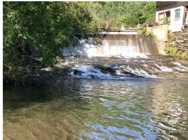
Hyde Dam site before removal (WRP)
