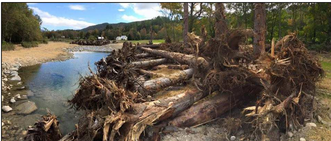
Photo 2 – Phase 1 engineered wood structure, looking downstream
