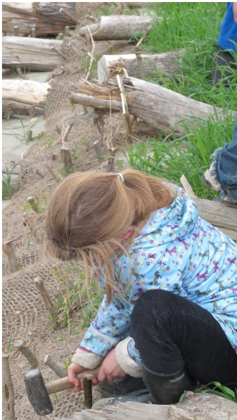
A Pomfret student pounds willow stakes in South Royalton. Each stake will grow into a lush and resilient willow whose roots will help stabilize the bank!
