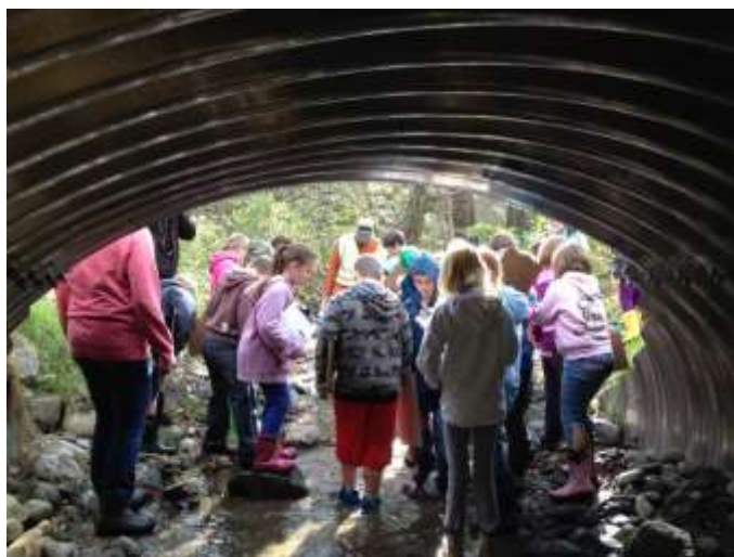
South Royalton 4 th graders measure and explore a newly-installed culvert on Broad Brook in Royalton (Emily Miller).
